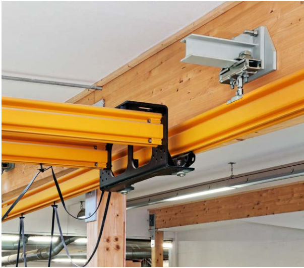
Rear-side anchoring of the support console to the laminated wooden beam.
